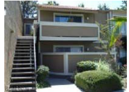
Bradbury Park Apartments
